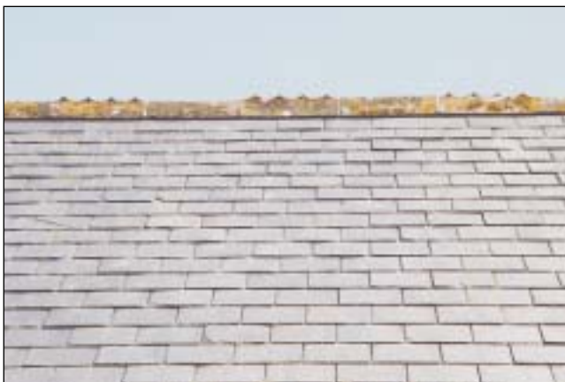
Above: Careful re-use of its ridge tiles has meant this roof has retained most of its historic interest and character even though the slates themselves required renewal. The appearance and hand-made qualities of the tiles are a positive asset.
