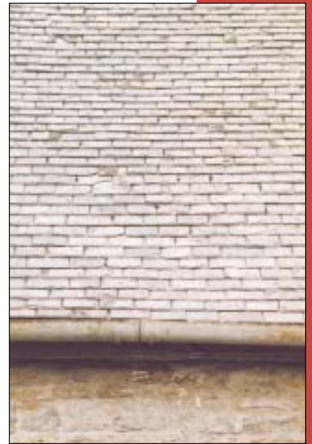
Right: Before the arrival of the railways, when mass-produced slates became available in abundance, all roofs were skilfully laid in this 'graduated' way.
