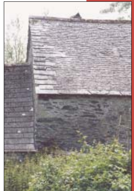
Right: As well as making the roof wind and weather tight, the larger slates at the eaves and verges create a very distinctive pattern.
