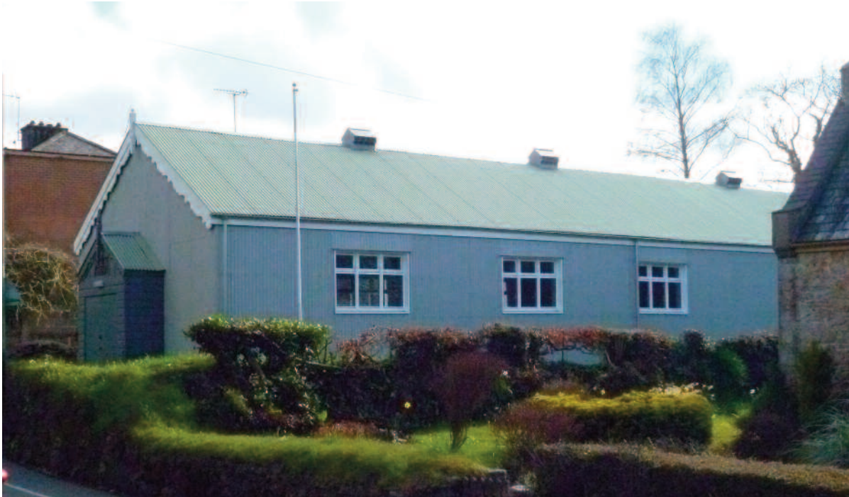
Dartington Village Hall - after refurbishment
