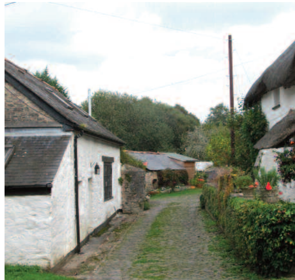
The former Youth Hostel at Lownard
